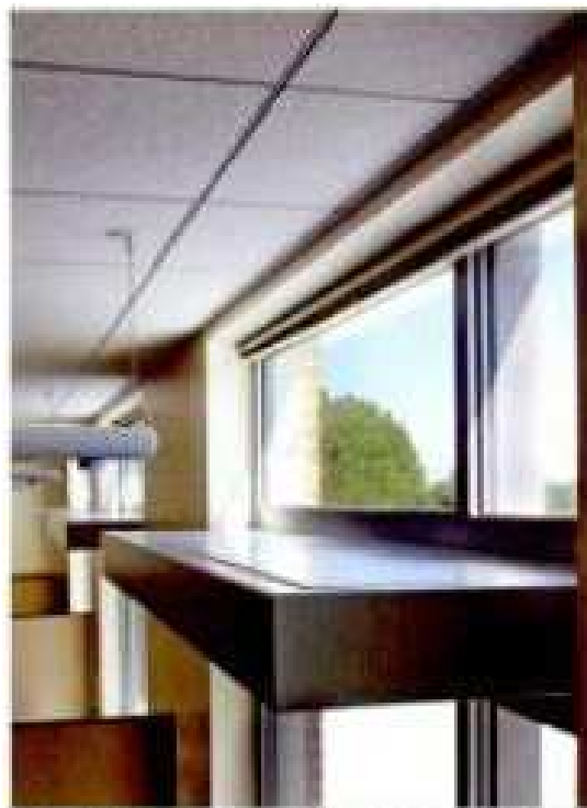
Figure 1: Light shelf bouncing direct light (LPA Architects,2009:28)
